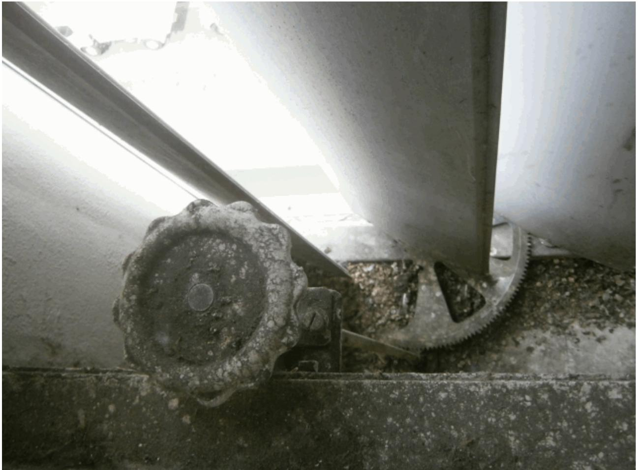
**Caption:** Internal detail of original aluminium louvre mechanism
